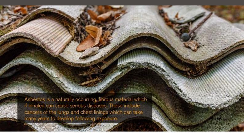
There are three main types of asbestos that can still be found in buildings today. These are 'blue asbestos' (crocidolite), 'brown asbestos' (amosite) and 'white asbestos' (chrysotile). All are dangerous carcinogens.
